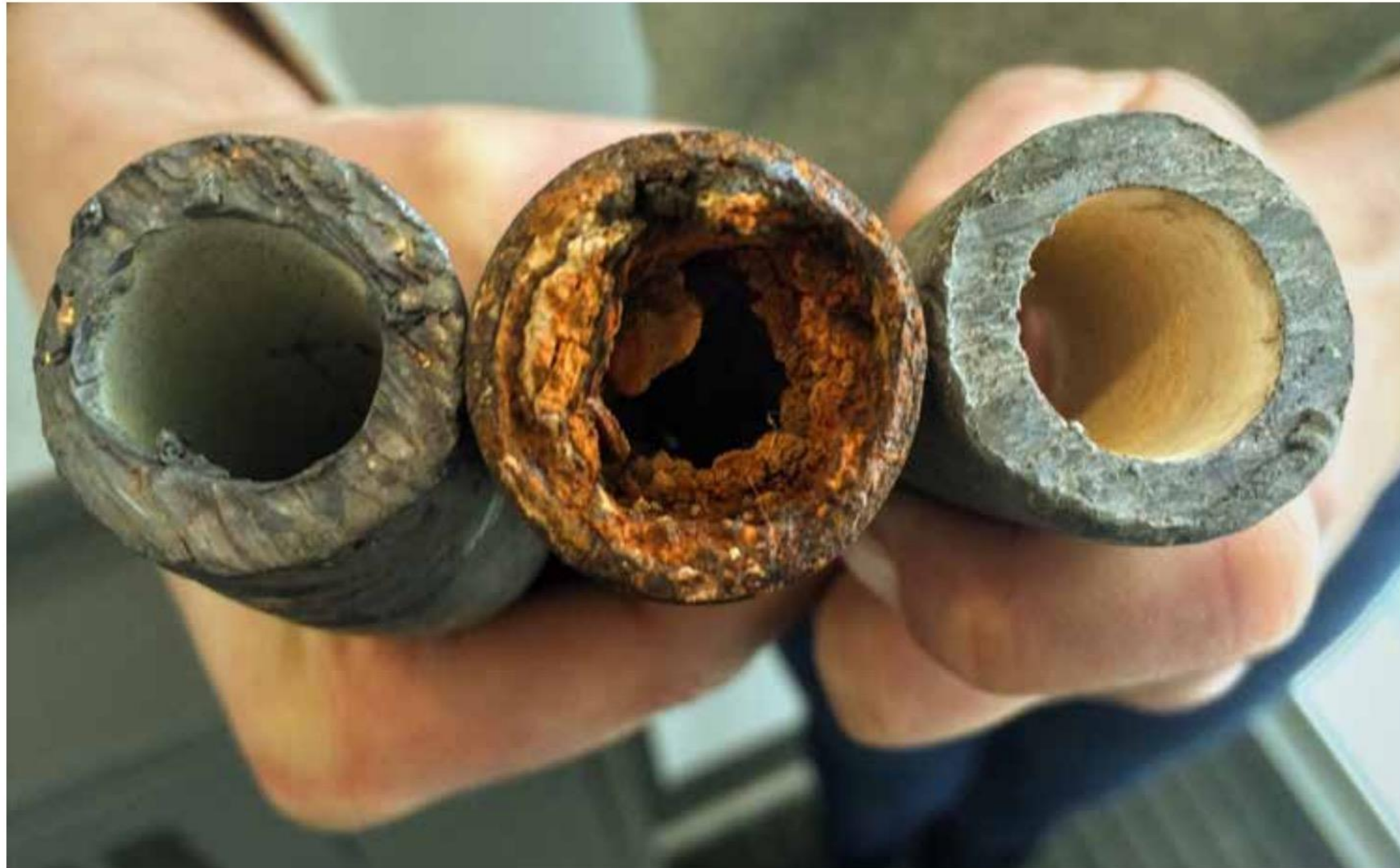
Pictured from left to right are a lead pipe, a corroded steel pipe, and a lead pipe treated with protective orthophosphate. Orthophosphate creates a film coating inside of lead pipes that can act as a barrier, reducing at least somewhat the amount of lead that gets into tap water.
